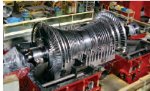
Steam turbine Tua-bin hơi
